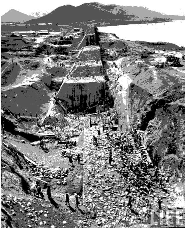
Fig 5.2 : Tungabhadra Dam Construction - 1952
